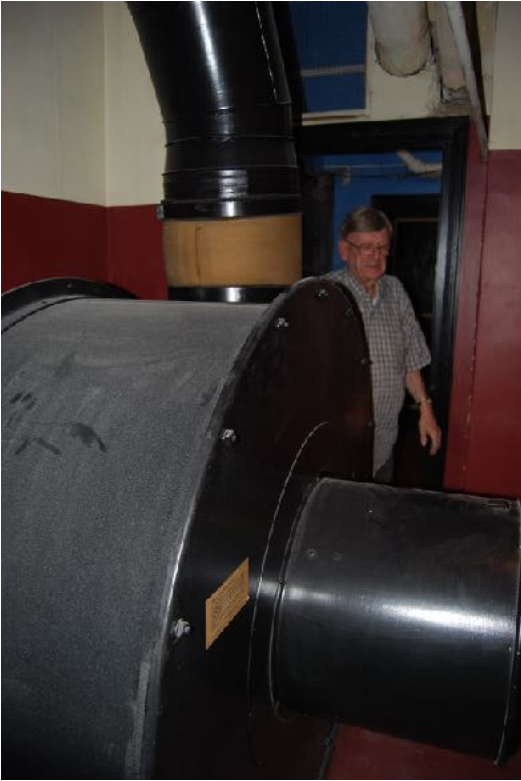
Working on the Robert Morton wind supply at the Warnors Theater
